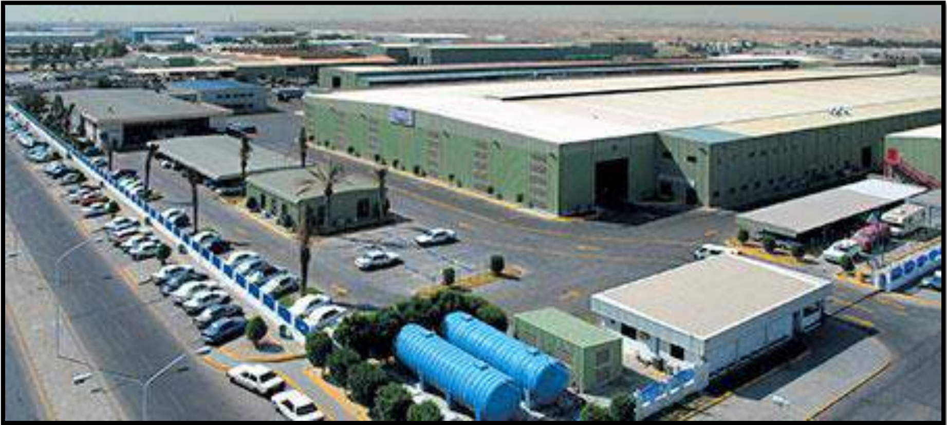
8,000 sqm of steel facility
